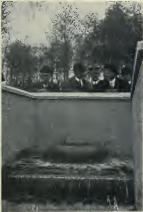
Discharge Chamber of Reservoir, at New Westminster.
